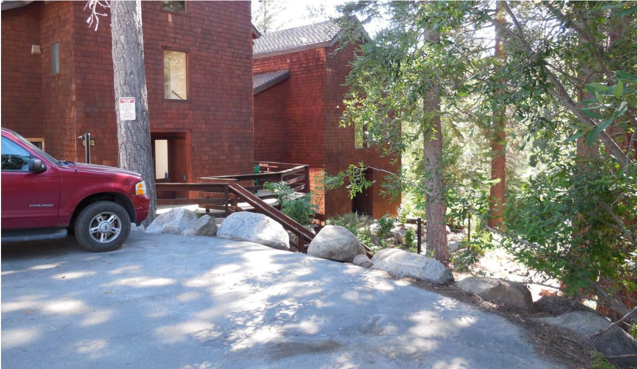
Location of 2-car Garage (photo take in July 2017)
